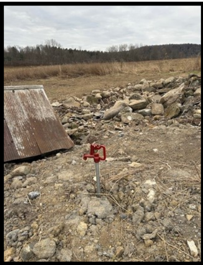
Above: Fence installed to increase rotational grazing Left: Hydrant installed off a spring development to add water to pastures Right: Access Road to gain access to pastures
